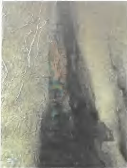
Cavity in the base showing decay in the stem.
